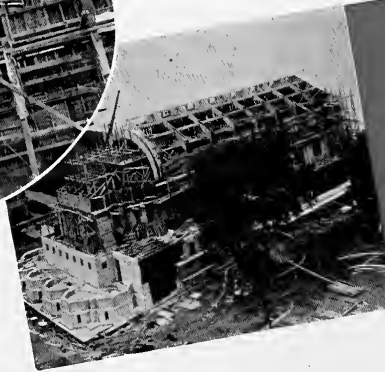
EARLY STAGES IN THE CONSTRUCTION OF THE CHAPEL.
